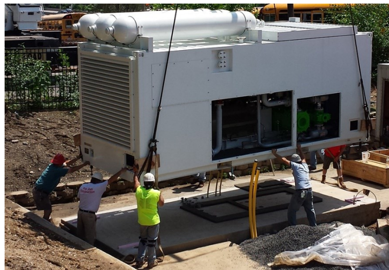
CNG Compressor Unit Installation
