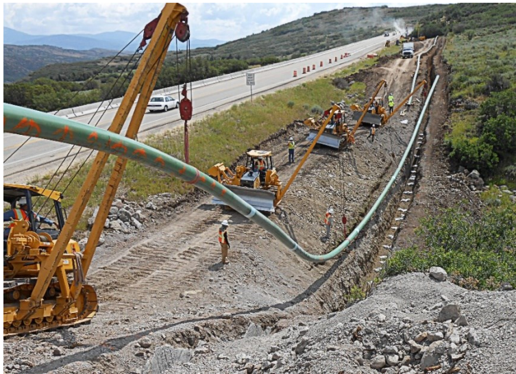
Natural Gas High Pressure 12" and 8" Pipeline Construction
