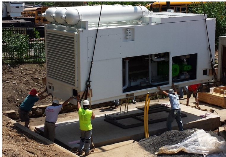
CNG Compressor Unit Installation
