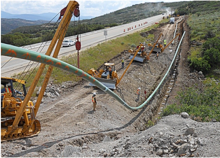
Natural Gas High Pressure 12" and 8" Pipeline Construction
